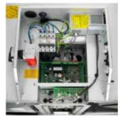
The easily accessible connection box with built-in switch disconnector and control system fuses ensures easy access for connecting and service.
