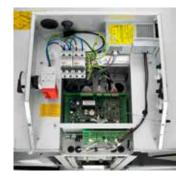
The easily accessible connection box with built-in isolator switch and control fuses ensures easy access for connection and adjustment. Read more about electrical connection in the guide "Electrical guide for
