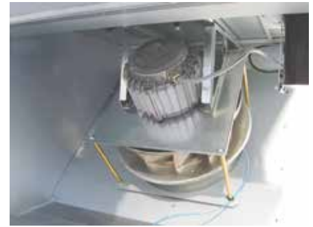
The motor sections are mounted in vibration dampers, which reduces noise in the ducts and eliminates the need to fit flexible connections between the unit and the duct system.
