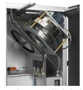
The motor sections are mounted in vibration dampers, which means less noise and vibration in the ducts, and there is no need to install flexible connections between the unit and the duct system. The motor sections are retractable for easier service. The motors are EC type with very high efficiency, meaning the requirements of the EcoDecian directions meeting the requirements of the EcoDesign directive.
