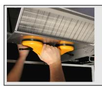
**EXHAUSTO** recommends: Handling of the heat exchangers is much easier with the vacuum lifter shown here.
